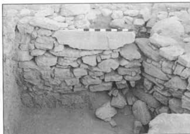
4. Area B, Square B2 western perimeter wall abutting the northwest corner tower, viewed from the east.
